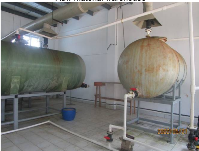
Raw material warehouse
