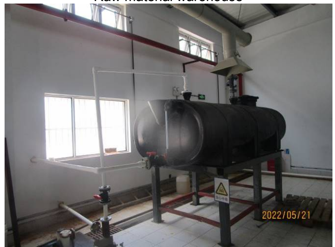
Raw material warehouse
